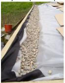
10. Fold underlay and polythene into gutter and staple neatly to top of lower cladding timber. Fill with pea shingle.
