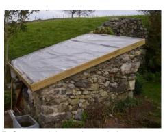
7. Cover with heavy duty polythene, loosely over the battens and staple a seam with the underlay to top of 2" 'lip'.
