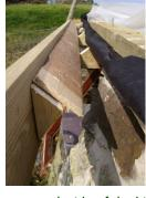
8. Fix slats to each side of the hidden gutter notches, ensuring that water will flow in the down pipe direction.
