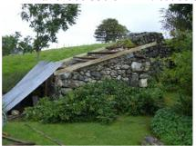
I. I used 3"x3" posts and 4"x1" cladding, fixed to the ends of the posts. The posts were firmly secured to the top of the stone walls with lime mortaring
