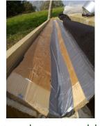
Use strong duct tape to seal the edges of the slats to the OSB board and bottom of the join. Add downpipe.
