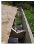
5. Cut V-shaped notches in battens extending below the Board and clad with 6"x1" as before. This will form the hidden gutter run for the roof.
