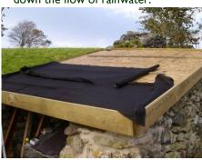
Cover board and battens with underlay and staple. Allow enough material to overhang edges.
