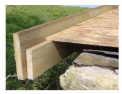
4. Fix 6"x1" cladding to the existing cladding timber. This will give you a 2" lip for soil and plant materials.
