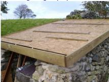
As the roof pitch is quite high, I fixed battens to the boarding to prevent the plant material from slumping. These battens will also catch and slow down the flow of rainwater.
