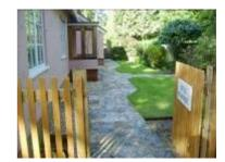
In the patio area, I made the patio slightly deeper by extending the leading edge to the outside wall of the extension. A brick soldier course gives a neat edge to the relaid limestone crazy paving. As I also levelled out the patio surface a little (and hid the manhole covers), this gave me an opportunity to add a lower step aligned with the kitchen door, echoing the new circular / rounded edges I had created.
